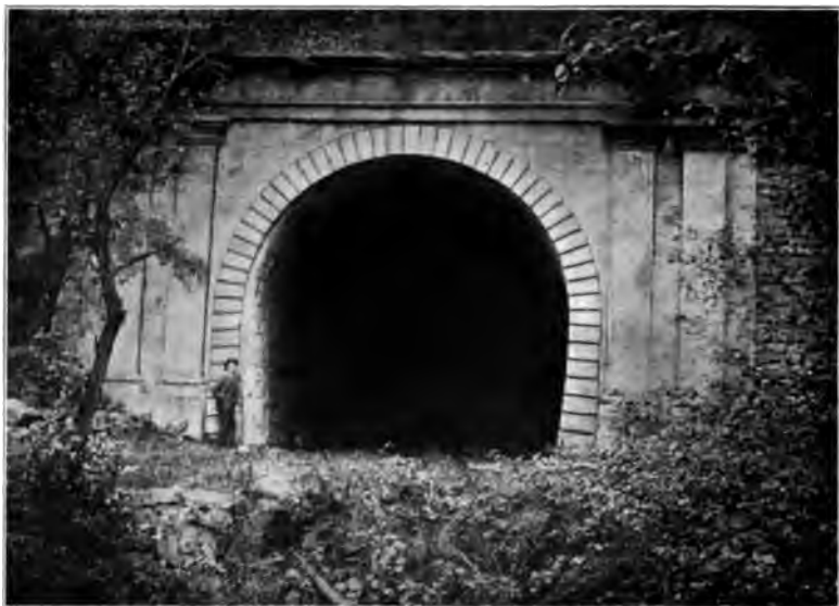
PORTAL OF THE ABANDONED TUNNEL OF THE ALLEGHANY PORTAGE RAILROAD NEAR JOHNSTOWN, PA., THE FIRST RAILROAD TUNNEL IN THE UNITED STATES
